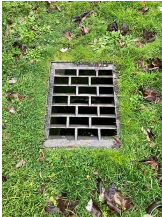
Picture 2: ROW on the west side of 2736 63 rd Ave SE Looking south
